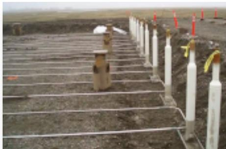
Thermosiphons installed at the Nikaitchuq oilfield on Alaska's North Slope, where they cool the ground and keep permafrost from thawing beneath a warehouse. Photograph: Courtesy of Arctic Foundation
